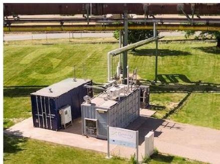
FuelCell Energy- rSOFC- SOFC 6kW/SOEC 32 kW
